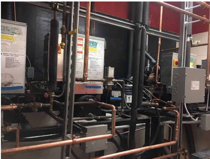
(a) new pipelines connection from condensers to cooling loop
